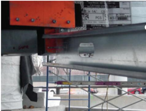
This picture shows the intersection of the RadiusTrack curved stud (on the left) with the structural framing (center). The single stud (foreground) is a typical crossbeam that spans between the curved ribs.
