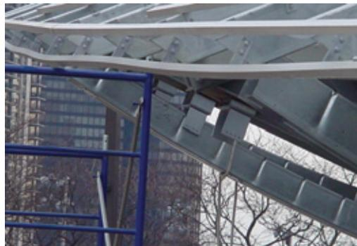
This sloped side face of the bridge is a ruled surface that derives its curvature from straight studs. The ends of the belly's curved beams are visible below and between the side framing. The intersection of the belly surface and the side surface are seen on the final pictures.
