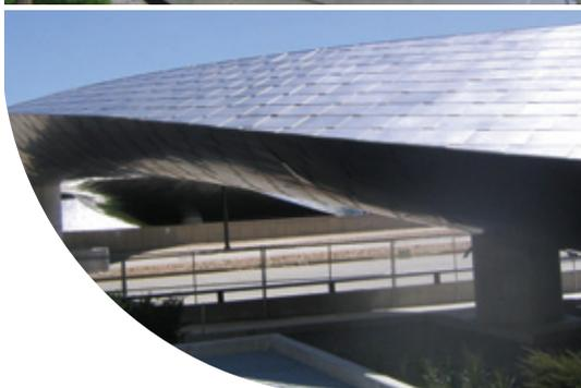
The studs in the skirt surface were flat, not curved. Clips that were attached to the studs took up the difference in the surface. With the simplified design, there were only eight different kinds of clips, each a different length, which were used for a dish in the surface.
