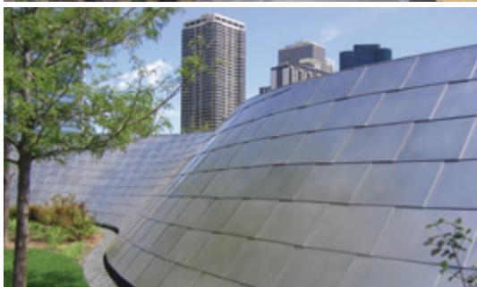
The Permasteelisa team ended up putting all of the variation into the stud. The aluminum panels and clips were all standard items that were fastened to the studs to create the curved surface. "We took one highly specialized component and a bunch of standard pieces and stretched a skin on it," said Harding. "Basically the skeleton made the shape."
